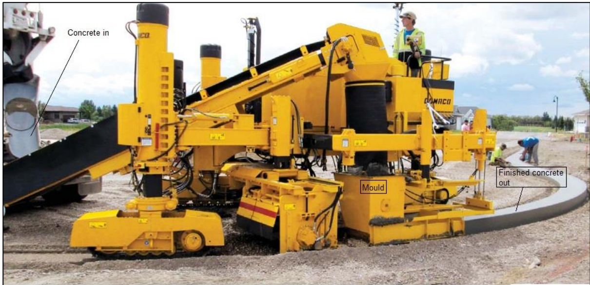
Diagram 2.4: Slipform Paver in Use on the Surface
