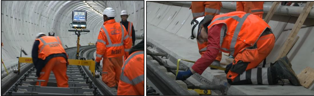
Diagram 2.16: Final Positioning of Rail
