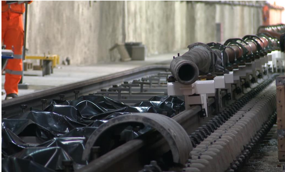
Diagram 2.18: Concrete Pump Line on Light Weight Wheels
