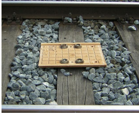
Diagram 2.8: Balise on a Wooden Sleeper
