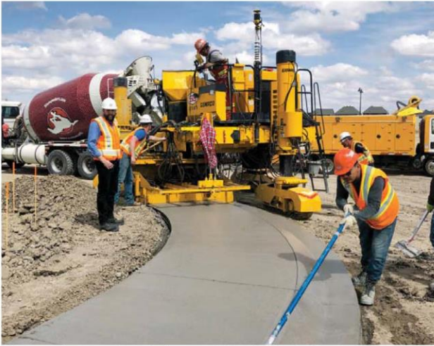
The three-track Commander IIIx slipforms monolithic sidewalk and curb and gutter.
