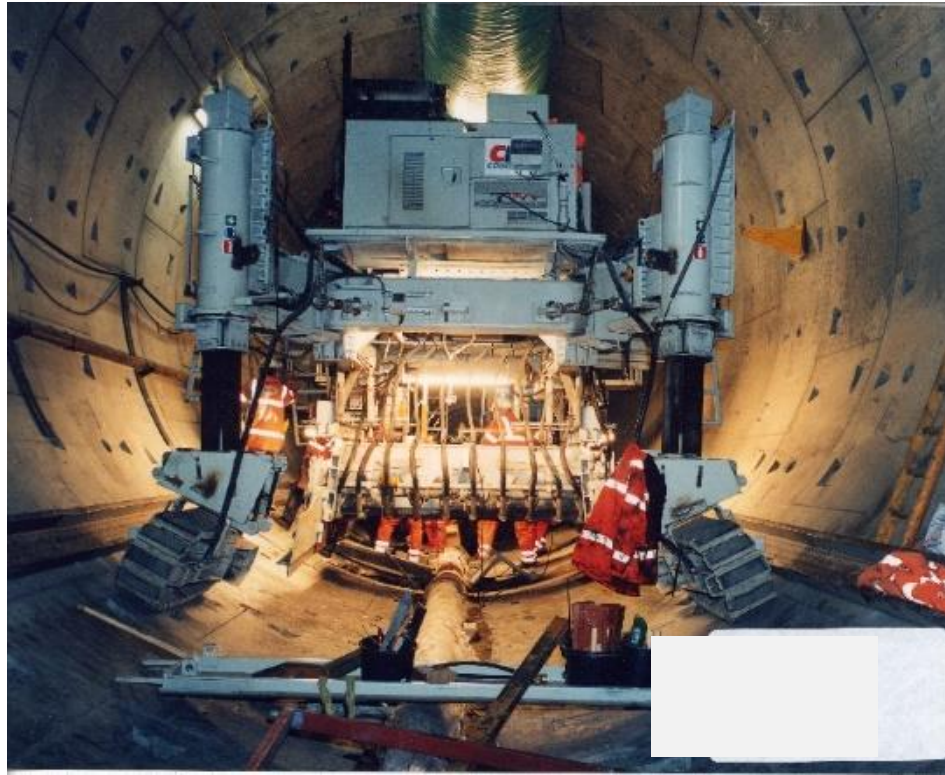
Diagram 2.11: Front of the Paver Where Concrete is Placed by the Excavator (Which is Behind the Camera)
